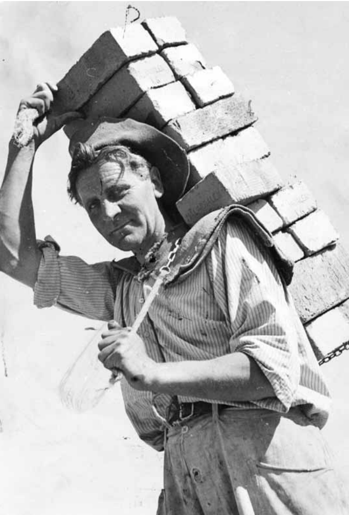
The building sector was in the past, and still is, plagued by accidents in the workplace. This 1945 poster shows a bricklayer shouldering a hod of bricks.
